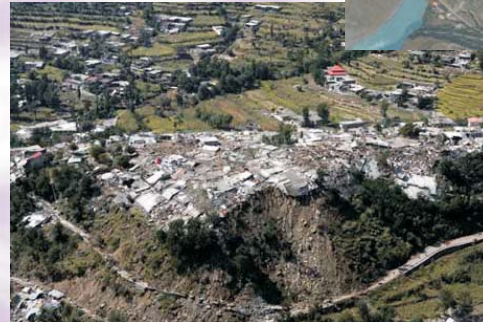
Mass Destruction in HFT Rupture Surface Zone, Balakot City, KPK, October 08, 2005 Earthquake
